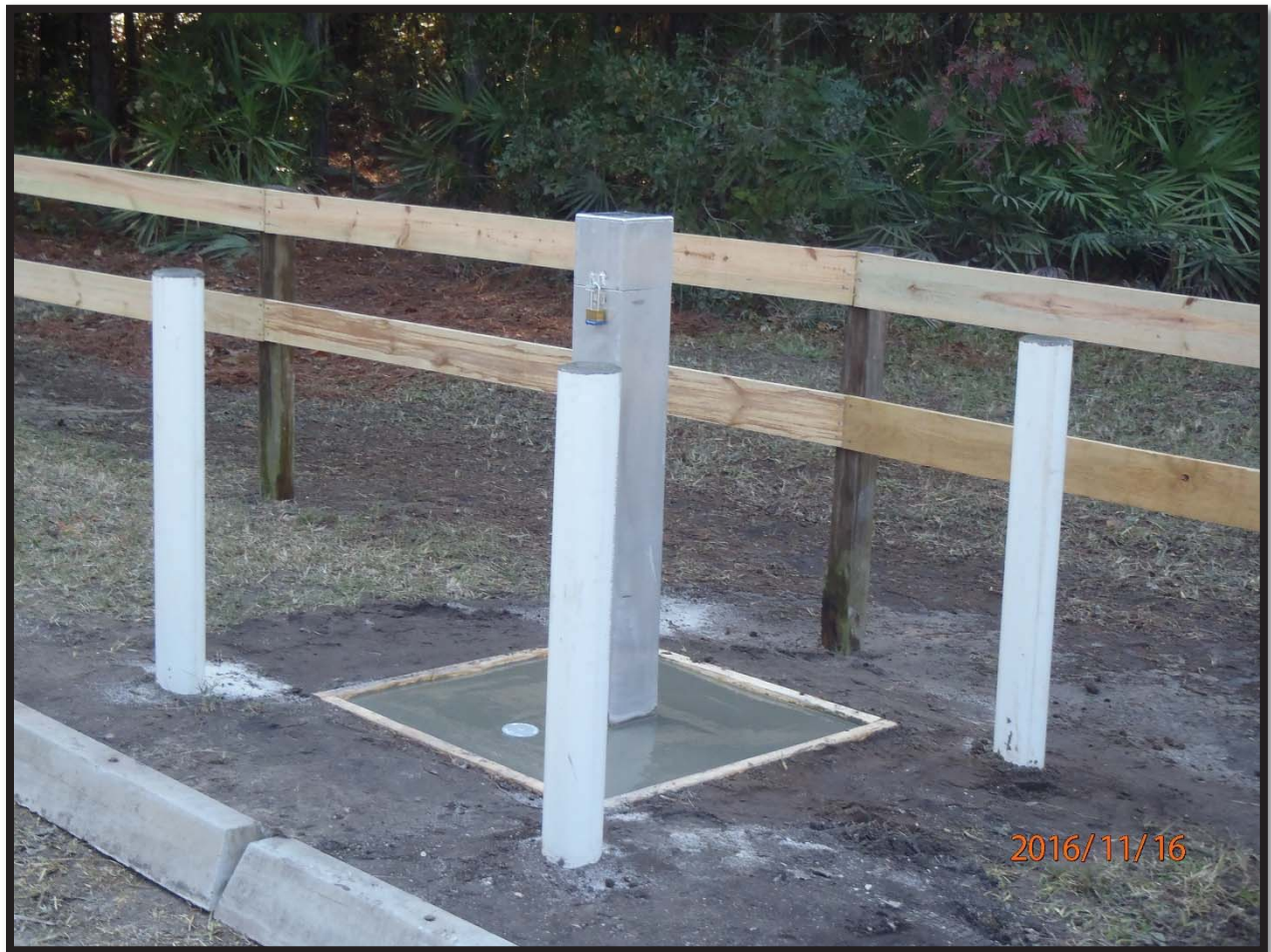
Figure 1. Completed Upper Floridan Well at Mill Creek North parking lot, Alachua County
