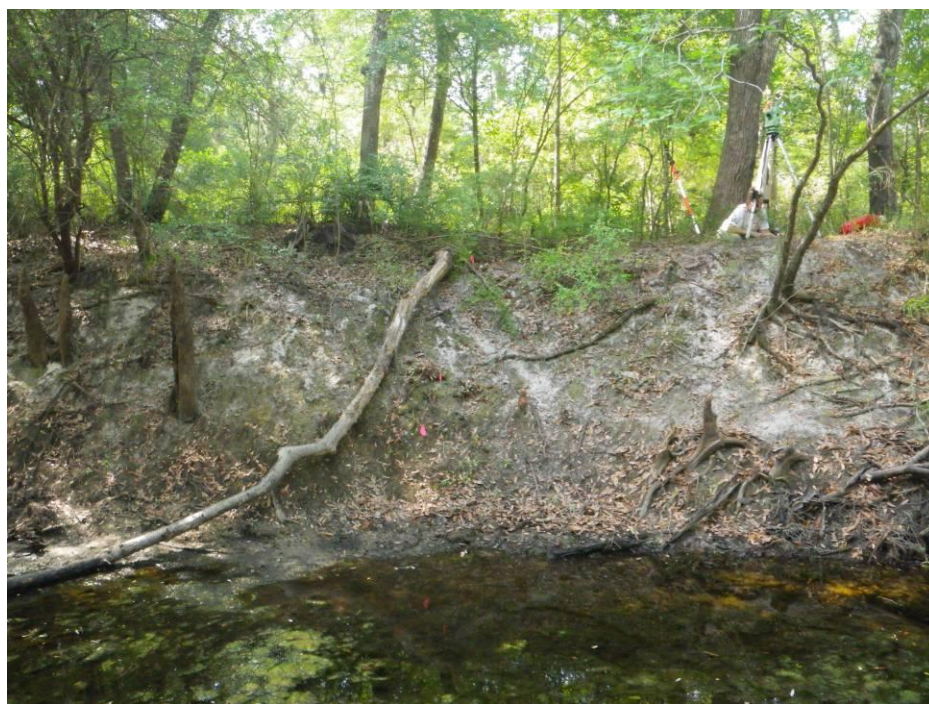
Photograph #8: Upper Santa Fe River – Worthington Springs XS-15 facing Left Bank
